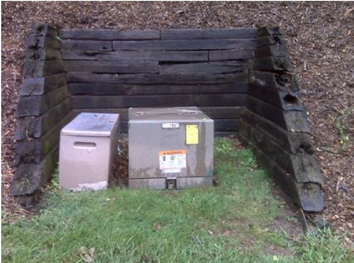
Figure 13.3 A Retaining Wall in Poor Condition
